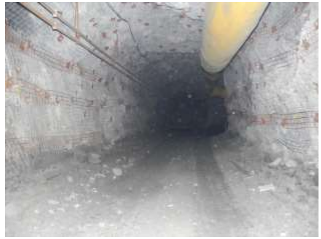
Low squeezing: rockbolts take load
