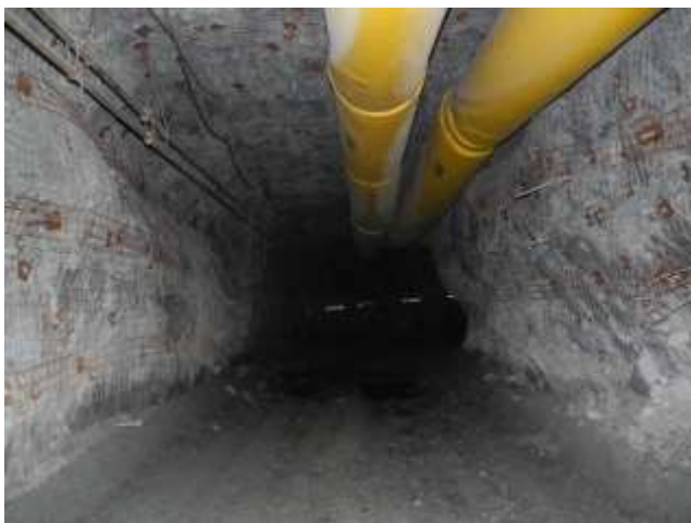
Moderate squeezing: convergence
