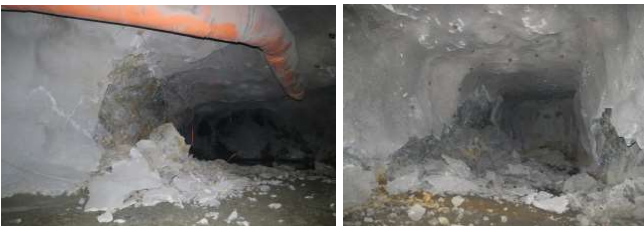
Figure 9. Examples of localised rockburst damage.
