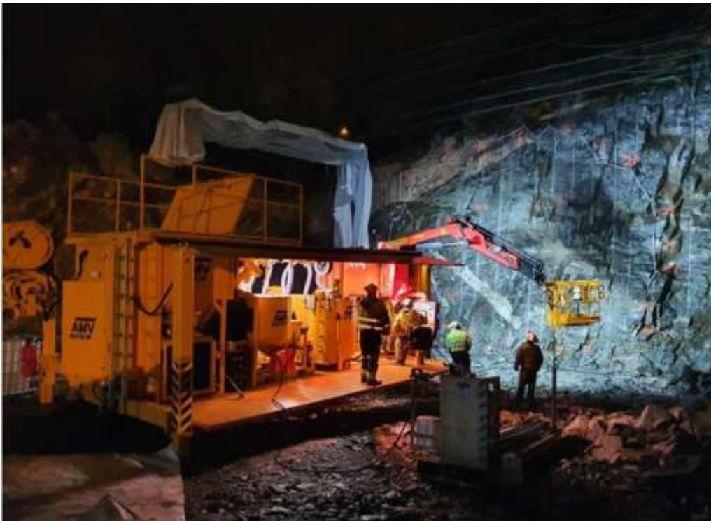
Picture shows preparations for pre-excitation grouting at Implenia/Acciona tunnel face in Moss. Picture by AMV
