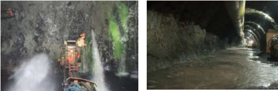
Figure 2. Inflow of 46°C hot water, total of 350 l/s.
